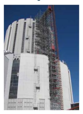
All HAKI stairs have a standard leg load capacity of at least 30 kN.
